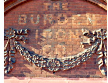
Burden Iron Works missing letters
